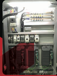
Automation (Extraction PPE 2 Renovation) 2023
