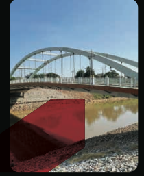
Construction of a bridge across the Nan River 120 m 2022
