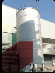
Fabrication and installation of Brew water tank No.2 2024
