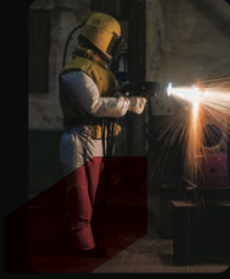
Thermal spray repair balancing block 2023
