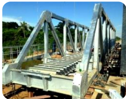
4. Rail Steel Bridge
