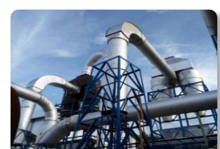
12. Duct & Stack Work
