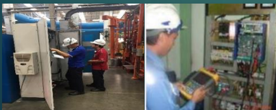
Manage and Supply Electrical Skilled Manpower-TCR
